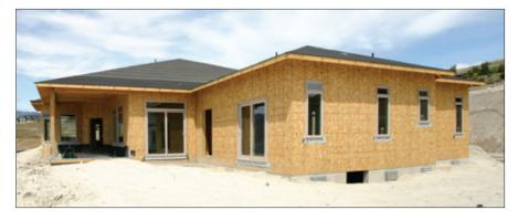
(APA Rated Sheathing); single-layer flooring (APA Rated Sturd-I-Floor®); and exterior siding (APA Rated Siding).
